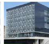
CIEM and CIRCE buildings Zaragoza (ES)
