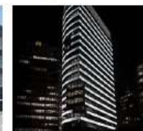
Raiffeisen Tower Vienna (AT)
