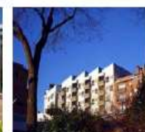
Meléndez Valdés and La Lliántia social housing buildings in Mataró (ES)
