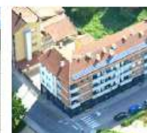
EspaZero office building Girona (ES)
